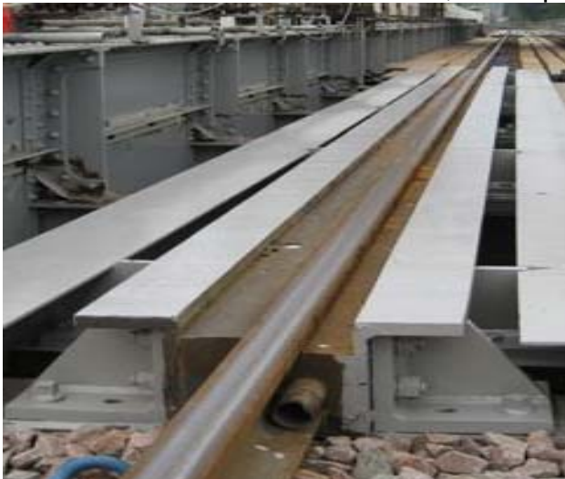
The Edilon Embedded rail system being installed.
