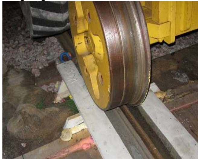
An RRV fitted with wide rail wheels derailing on the Edilon Embedded rail system
